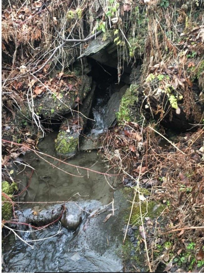
Hollyhock Culvert: Outlet
