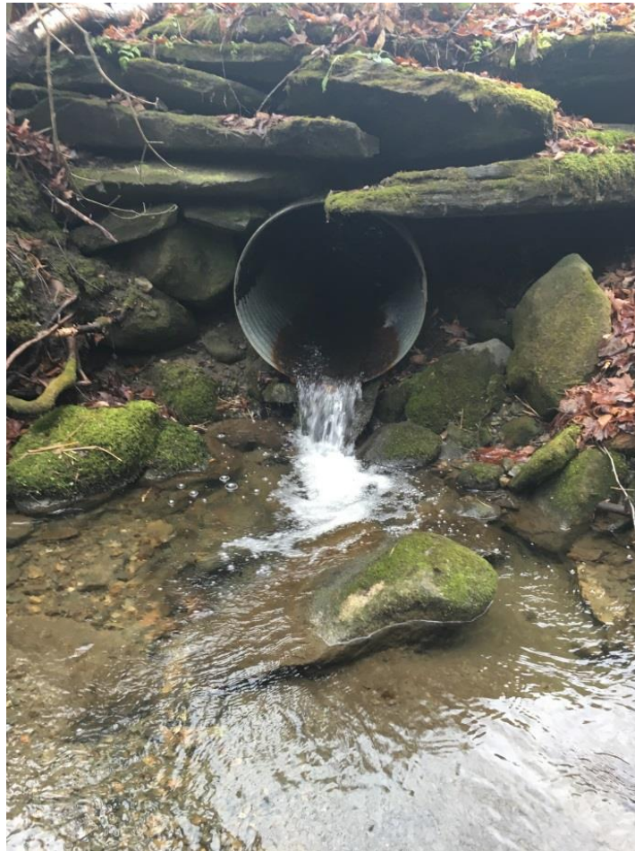
Peth Road: Culvert Outlet
