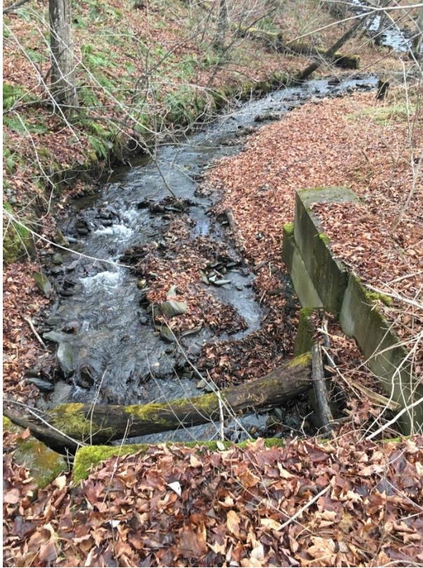
Brainstorm Road: Culvert Outflow
