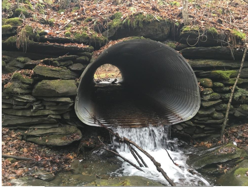
Farnsworth Brook Road Culvert Outlet
