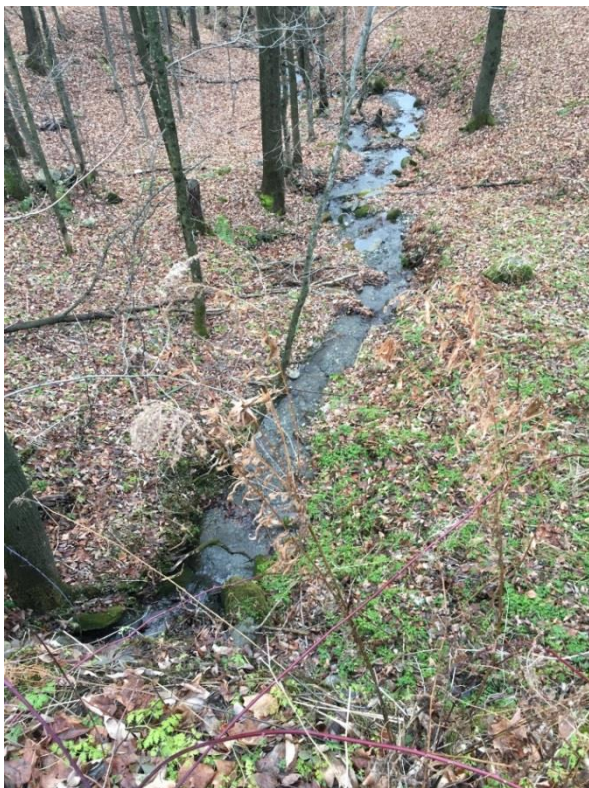
Peth Road: Culvert Outlet Stream
