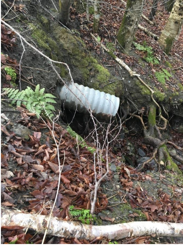
Peth Road: Culvert Outlet
