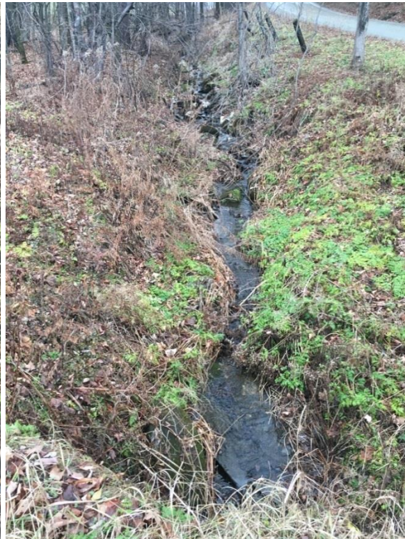
Culvert at the Junction of Peth and Brainstorm Roads: Inlet Stream
