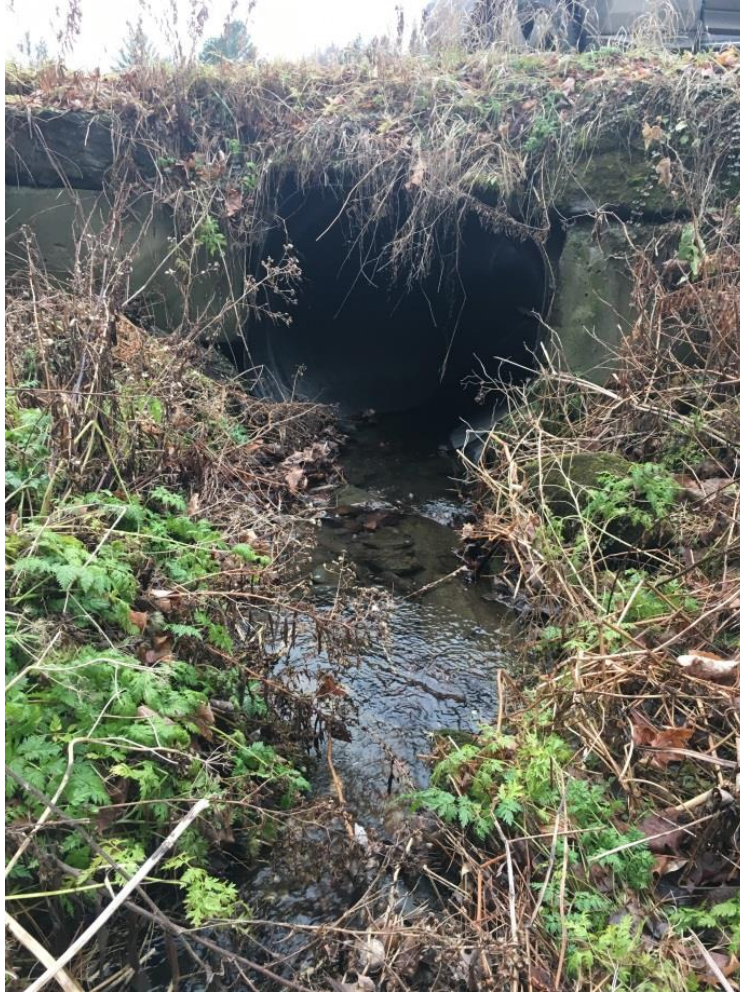
Culvert at the Junction of Peth and Brainstorm Roads: Outlet
