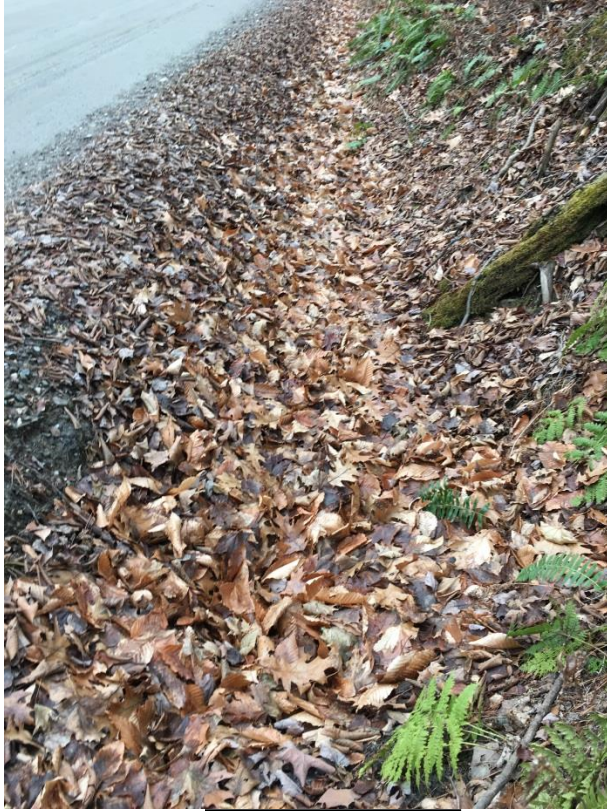
Ditch at Inlet
