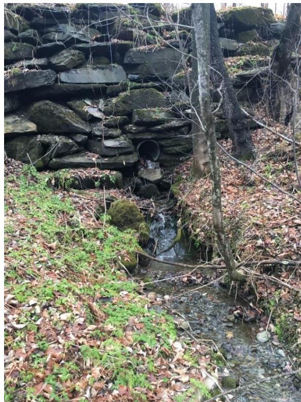
Peth Road: Culvert Outlet and Rock Wall
