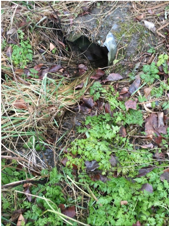
Peth Road: Culvert Inlet
