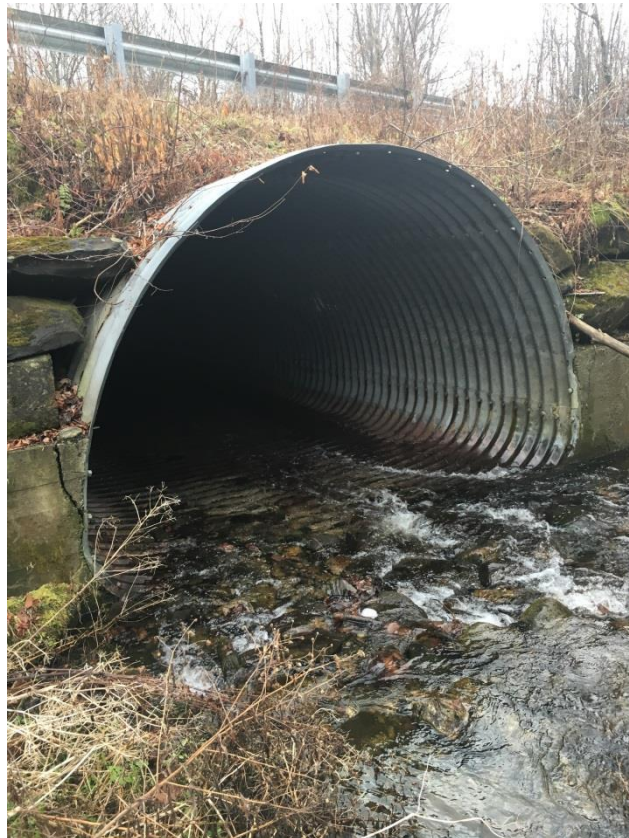
Culvert at Junction of Peth and Labounty Roads: Inlet
