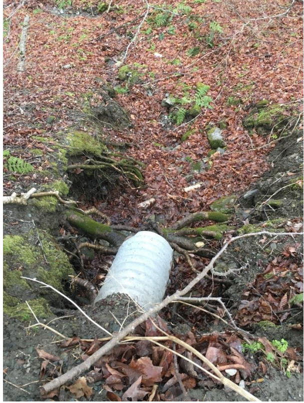
Peth Road: Culvert Outlet
