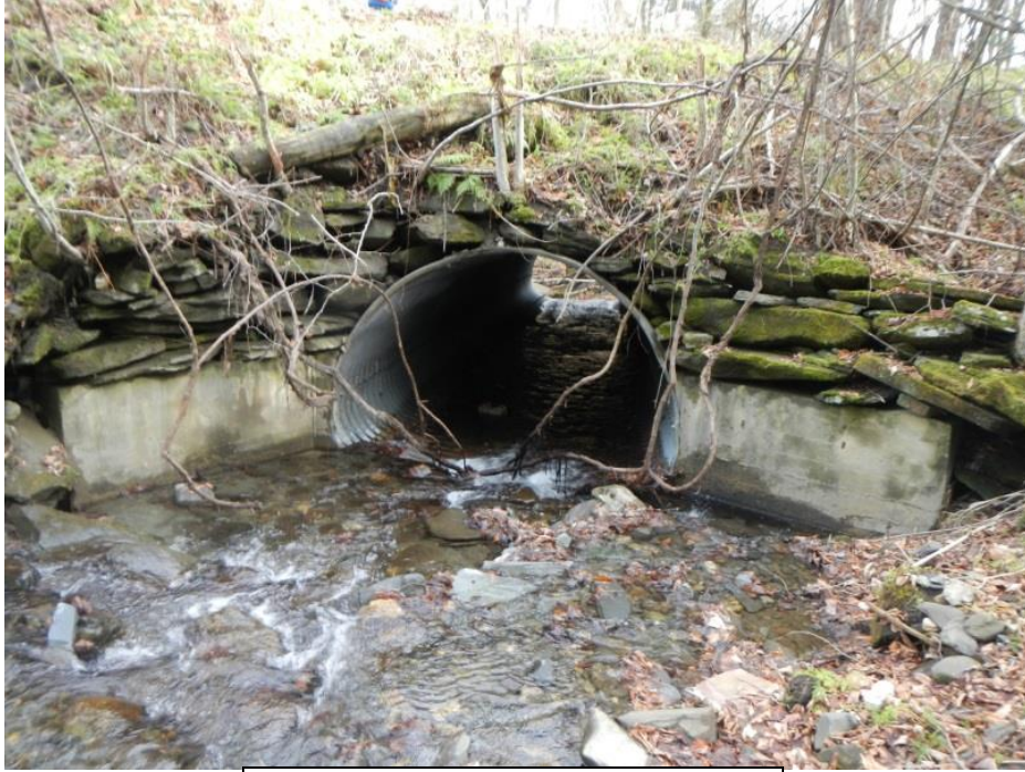
Farnsworth Brook Road: Culvert Inlet
