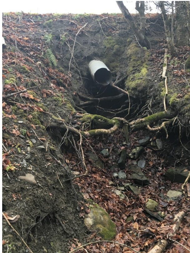
Peth Road: Culvert Outlet
