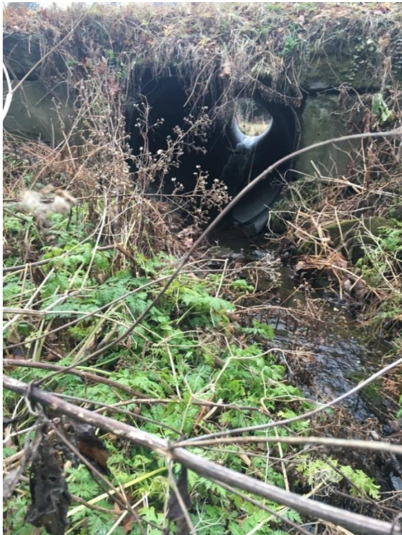
Culvert at the Junction of Peth and Brainstorm Roads: Inlet
