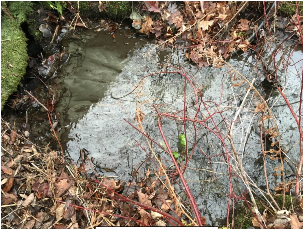
Hollyhock Culvert: Inlet
