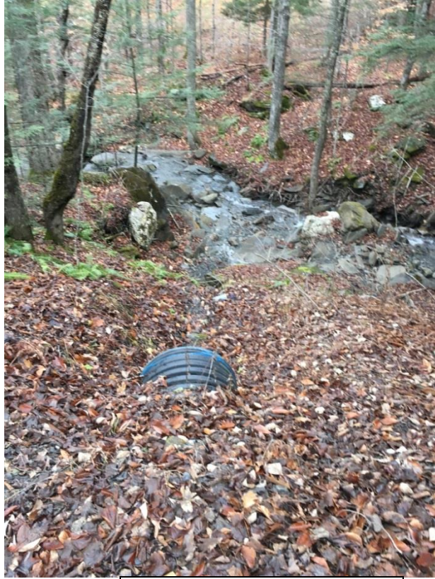
Culvert discharges to surface
